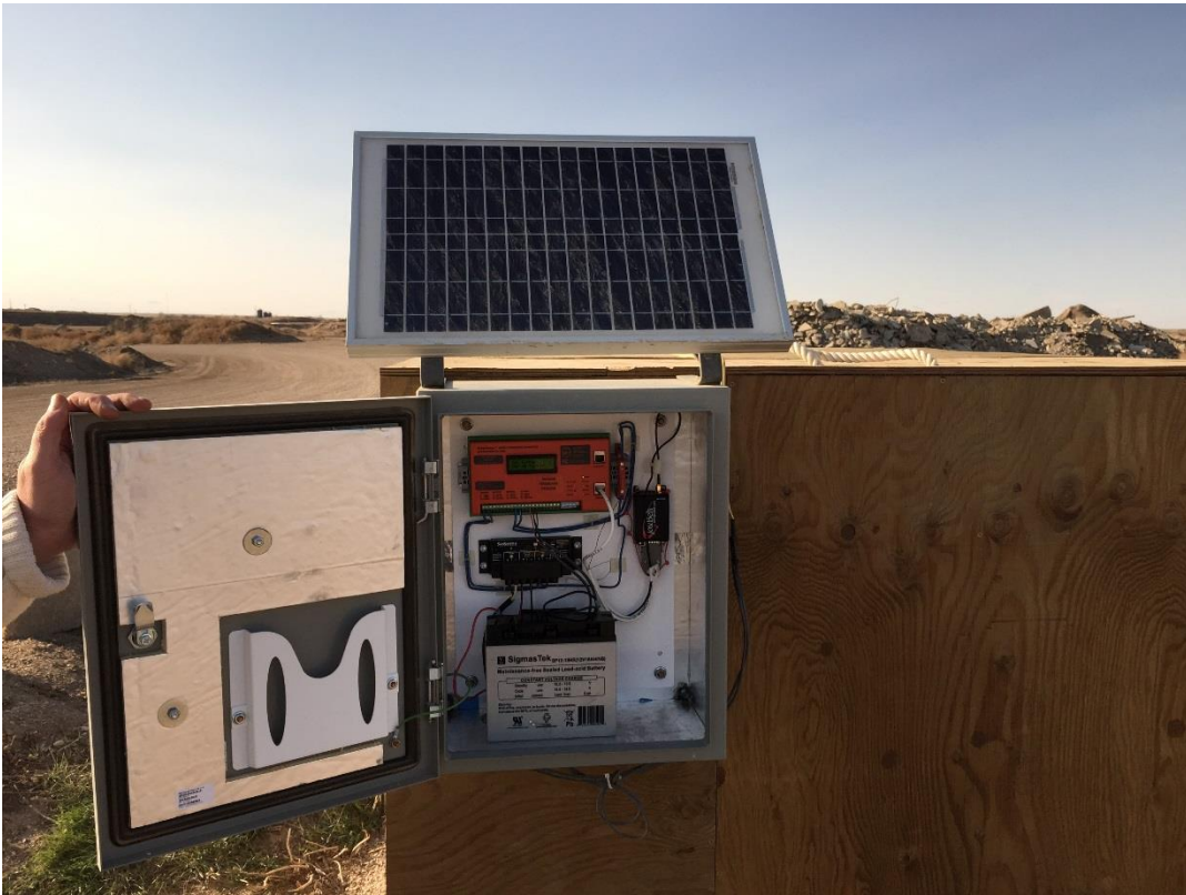
EtherMeters Installed as part of a Satellite-Based, Frac Water Automatic Metering System. (Near Williston, ND)
