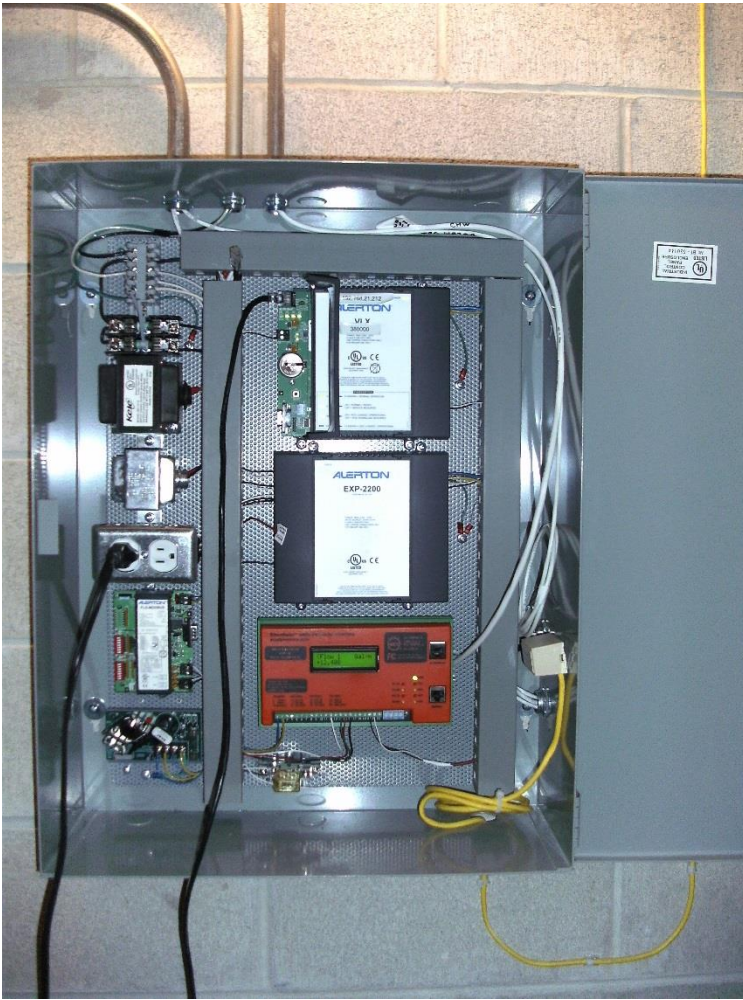
EtherMeters Installed as part of a University Building Automation System. Illinois Institute of Technology (Chicago, IL)
