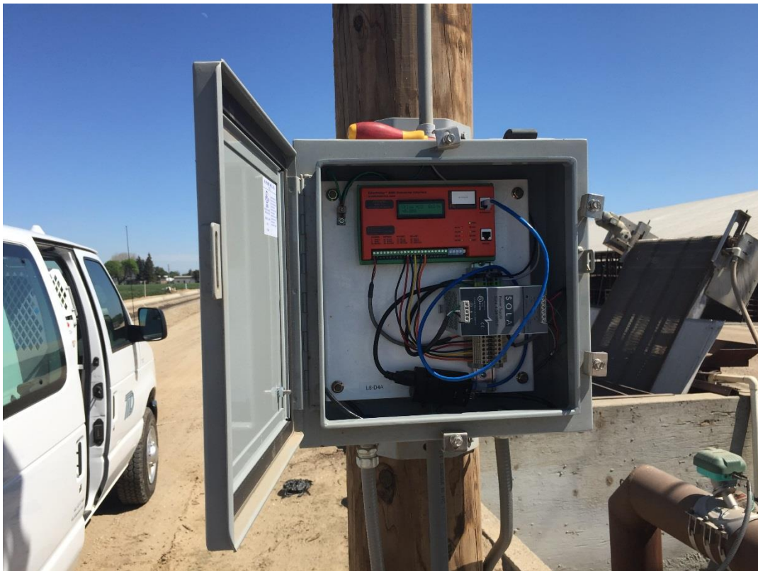
EtherMeters Installed as part of an Irrigation Monitoring System. Turlock Irrigation District (Turlock, CA)
