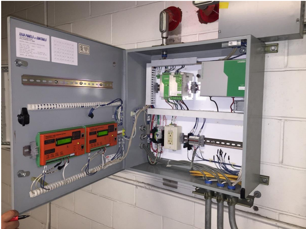
EtherMeters Installed as part of an Airport Energy/Utility Management System. JFK International Airport (New York City, NY)
