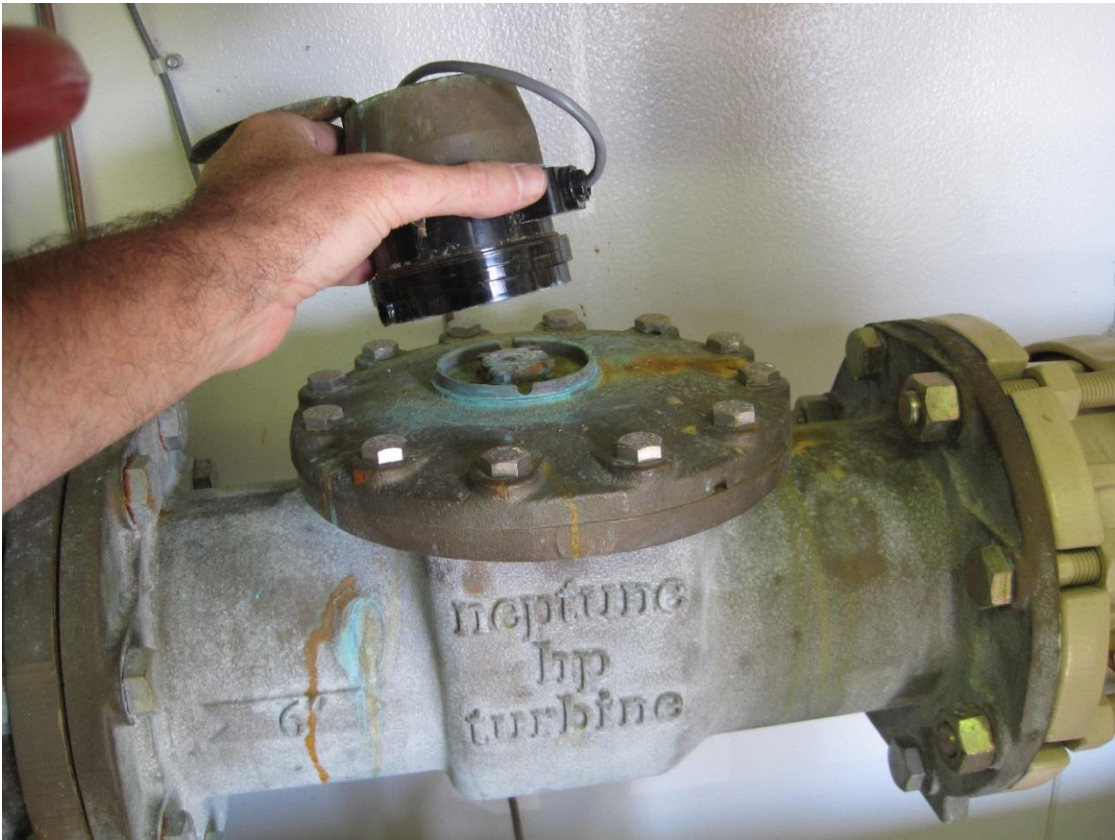
Removal of Direct-Read Register and Tricon/E3 Instrument
