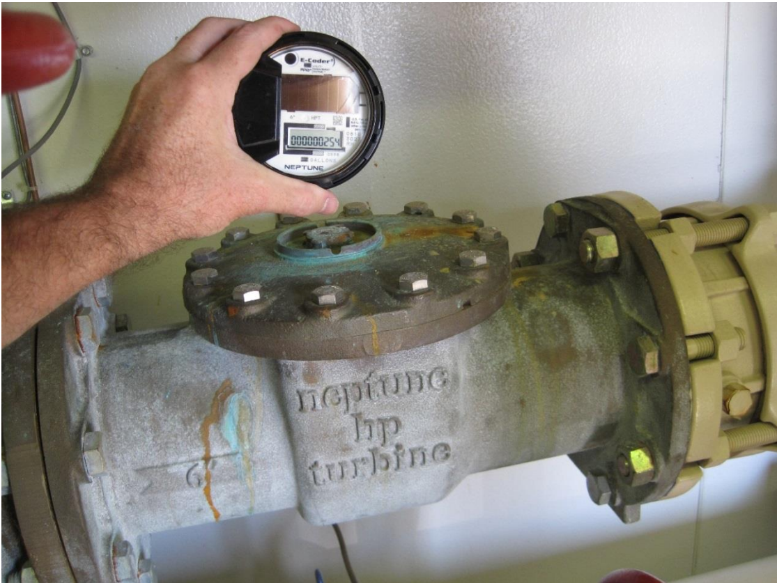
Neptune E-Coder Register (Absolute Encoder), Pre-Installation. Note - Also works with Neptune Pro-Coder Register.
