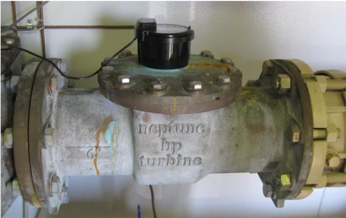
Neptune 6-Inch High-Performance Turbine Meter, with E-Coder (Absolute-Encoder) Register
