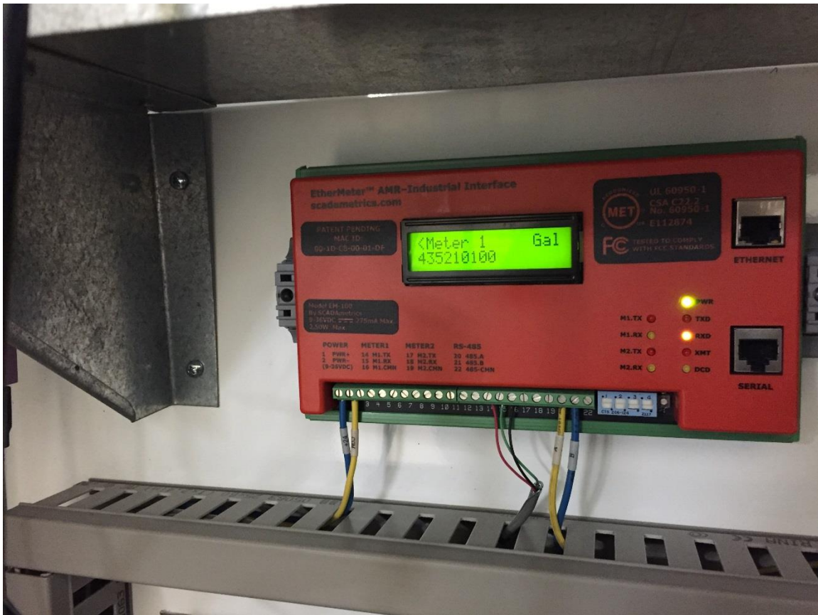
SCADAmetrics EtherMeter, Flow Meter Gateway Between Sensus 6 Inch Omni-T2 Meter and SCADA System. SCADA Connection Medium: Modbus/RTU (RS-485). Note the Perfect Agreement Between the SCADA Totalizer and the Omni Meter's Totalizer!
