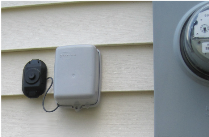
Left: The TRF-W Provides Water Utilities With The Flexibility Of Reading Meters Using Either An AMI Radio Endpoint or a Touch-Read Pad.
