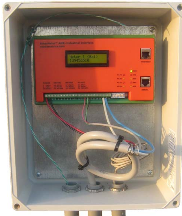
An Installed EtherMeter™ AMR-Industrial Interface
