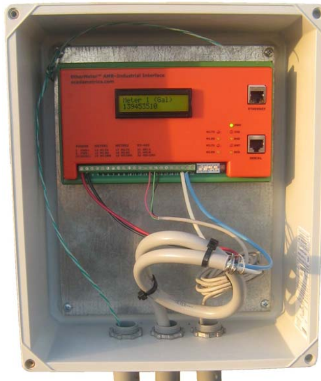
An Installed EtherMeter™ AMR-Industrial Interface
